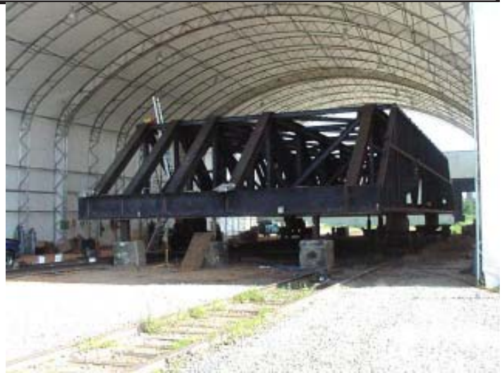
Steward Machine, Birmingham, AL uses the Meta-Lax stress relief equipment for post weld stress relief of this 480,000 lb overhead lock door. The door is part of the U.S. Army Corps of Engineers Olmsted Lock and Dam Project on, Ohio River.
